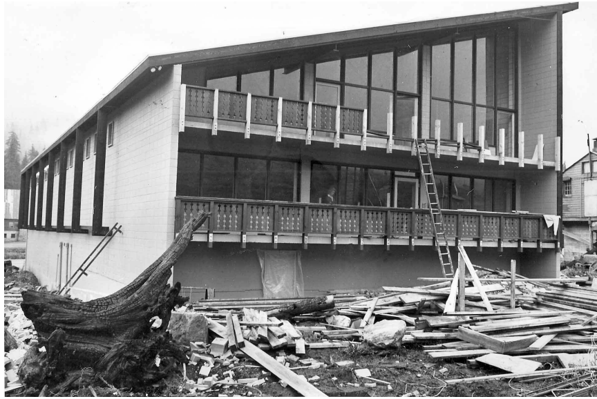
Lodge at Snoqualmie Summit under construction. Courtesy of the Moffett family.
