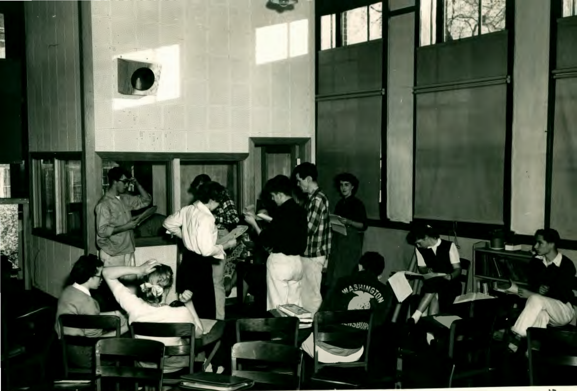
Classroom with Radio Broadcasting Booth in Rear, Senior High School
