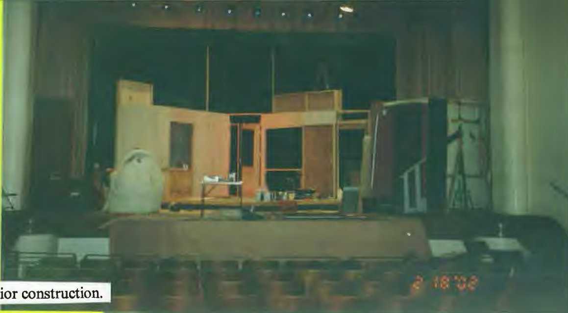
Interior and Plant #4 construction.
