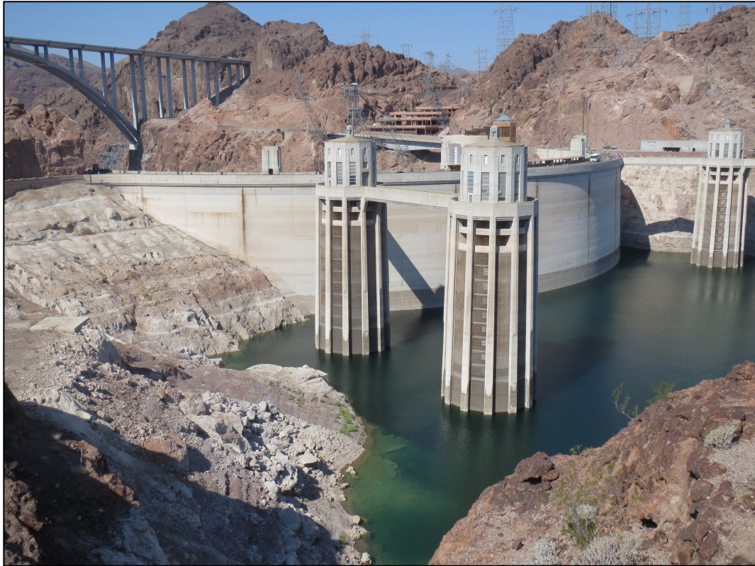
Figure 6 Drawdown at Lake Mead, the nation’s largest reservoir, in 2014 ( source : photo by author ©2014)
