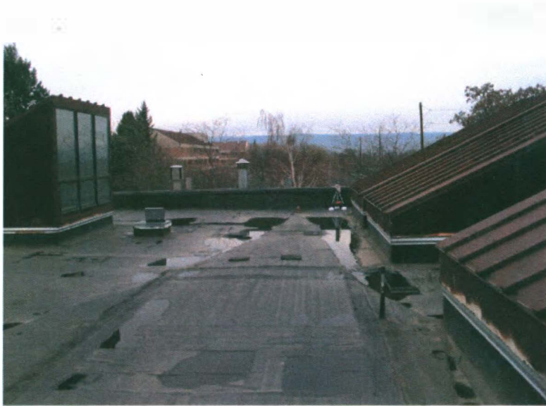
Figure A1. Setup photograph of Location 1 (Randall Hall) roof.
