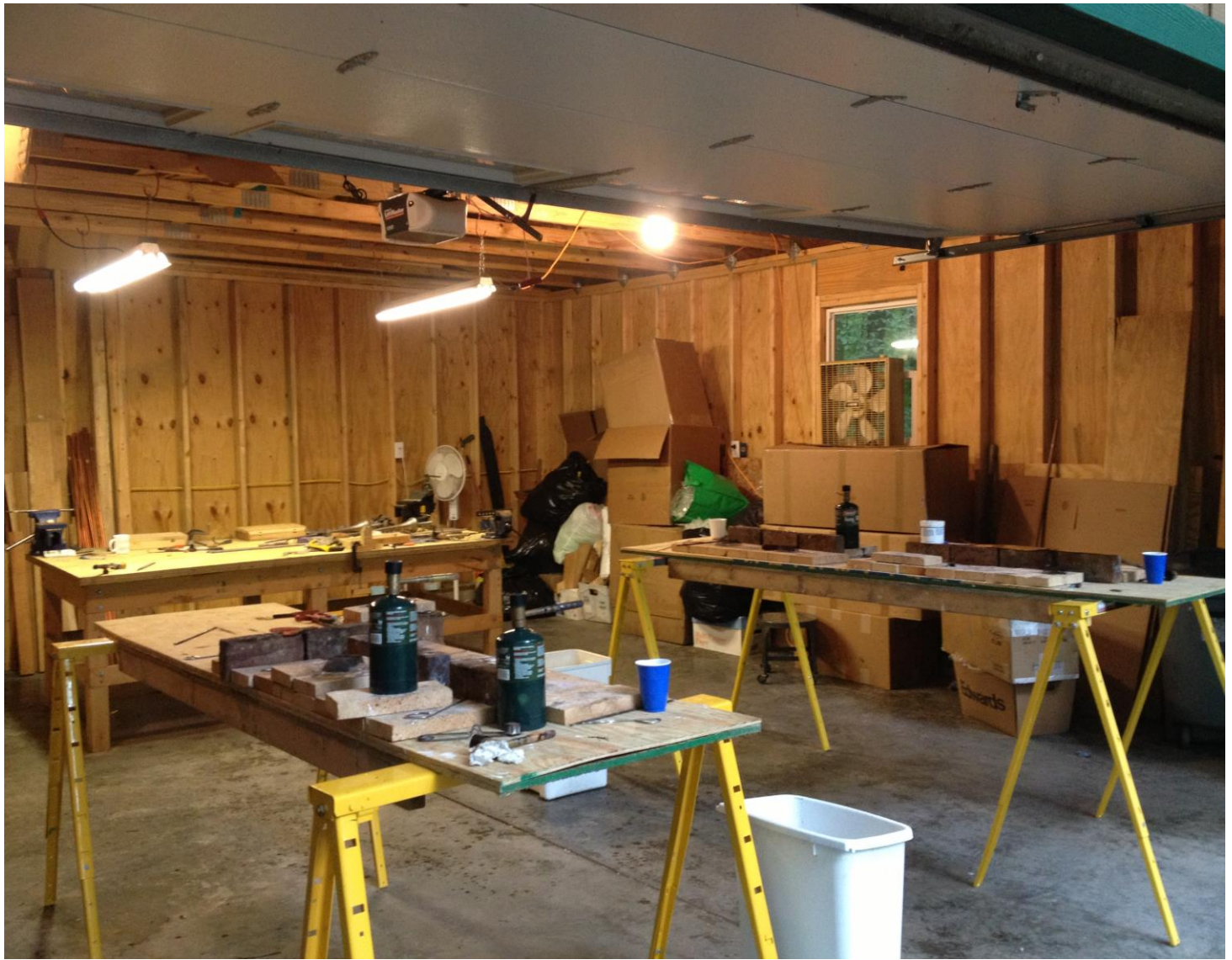
The garage with multiple soldering stations
