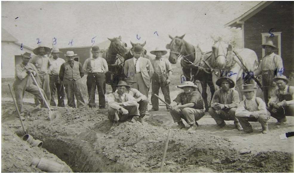
Figure 71. Putting in Moxee City water. Everyone in town helped. Date unknown. (Barbara Beane Photo Collection, Yakima Valley Museum, n.d.).
