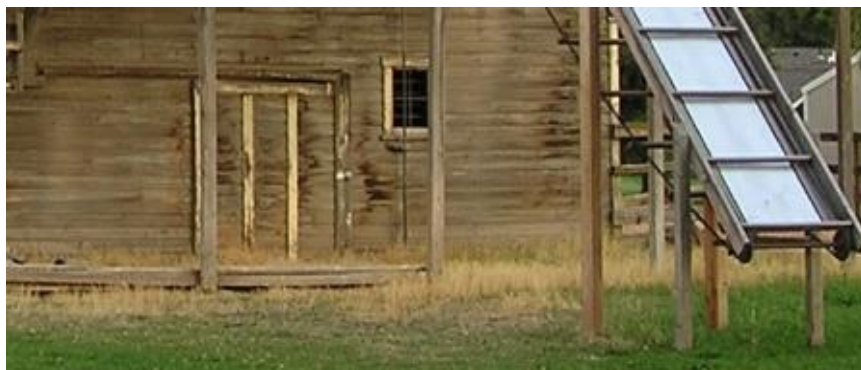
Figure 108. The furnace or drying ovens are behind the sliding door. Slab wood was usually stacked high during hop harvest, making the doors difficult to see.
