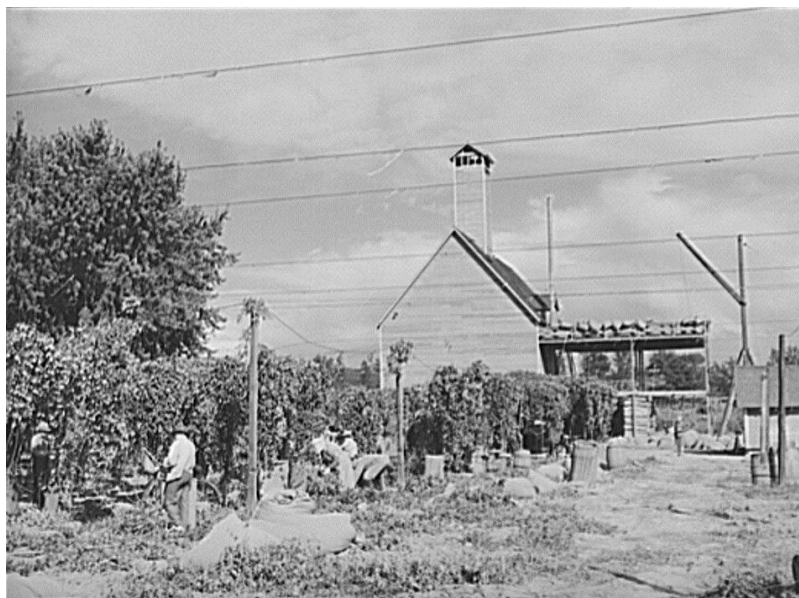
Figure 151. Hop pickers. Yakima County, Washington. Single hop kiln similar to the Gendron Ranch kiln. Hop yards with people picking. Notice this hop yard is not that tall. They are picking into baskets, and the kiln is heated with slab wood as seen under the deck loaded with sacks of green hops. Russell Lee, 1941. Photo may be later than this date.
