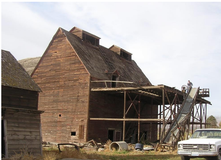
Figure 104. Paul Patnode Hop Kiln on Faucher Road, Moxee. It is a double kiln with two cupolas. (Terri Towner, 2010).
