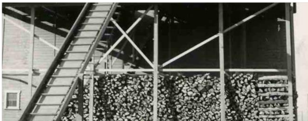
Figure 76. Hop elevator with slab wood in the background. The elevator on the left, runs from ground level to the deck of the kiln drying room. Slab wood is stacked in front of the doors, to the kiln furnaces, that dried kilns of freshly lain hops. (Gendron Photo Collection, 1920)
