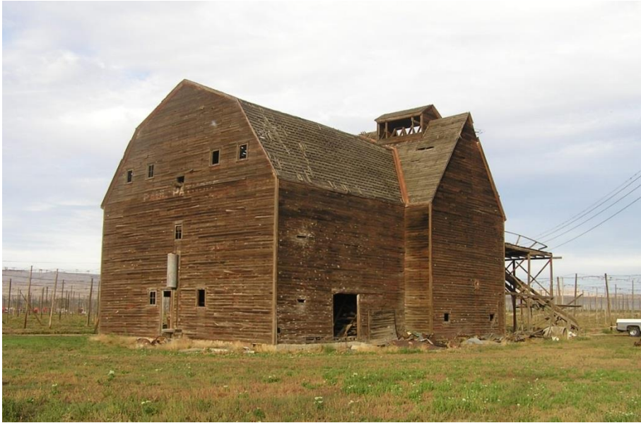
Figure 110. Southwest view of the Paul Patnode Hop Kiln. (Terri Towner, 2010).
