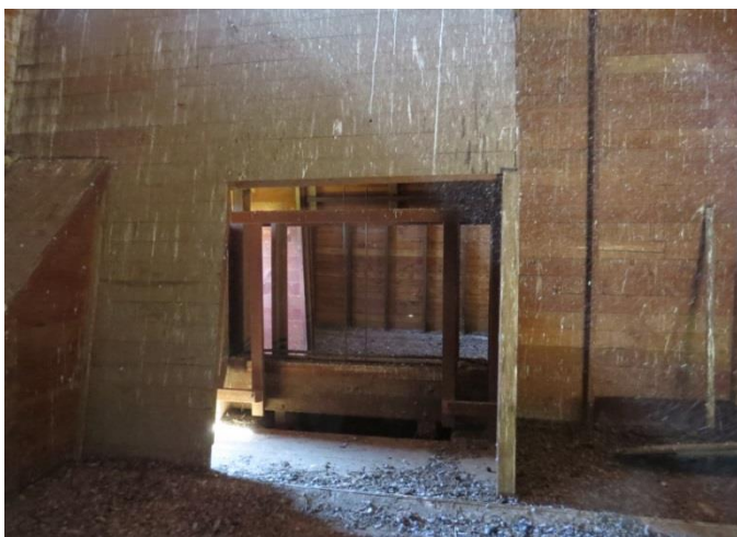
Figure 126. The doors to the press are open on both sides in the cooling room. In this picture, the press is fully extended to the first floor main baling room. Two people would shovel the cooled hops into the shoot. Ken and Russ Duffield would take this job at the Gendron Ranch each evening after finishing their dairying chores (Terri Towner, 2016)
