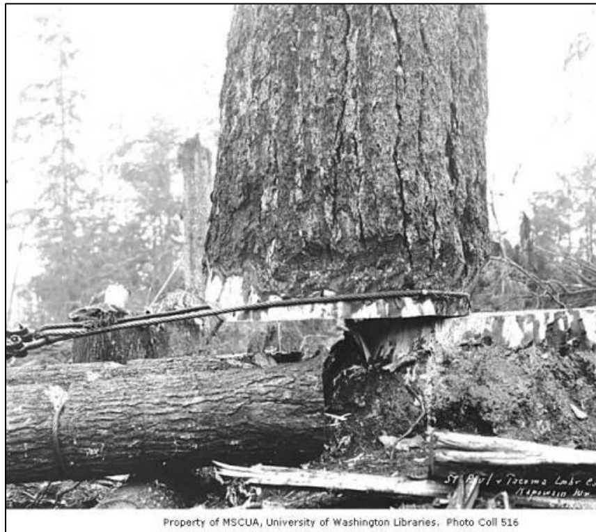
Figure 6. Undated photograph of the base of a spar tree worn down by cables used during SPTLC logging operations in Kapowsin, Washington (C. Kinsey 2017h).
