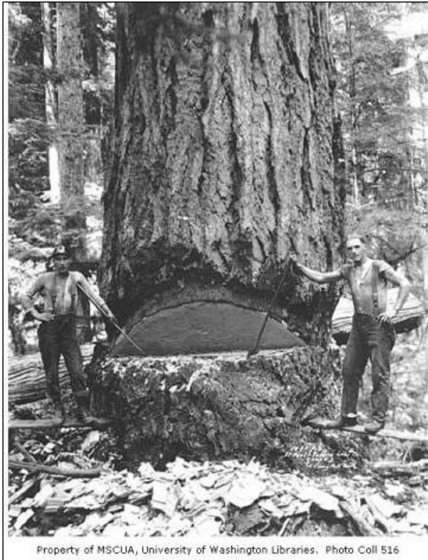
Figure 15. Photograph of SPTLC employees, from Camp #3, cutting down a 10-foot-wide fir tree near Orting, ca. 1926. Note the use of springboards and double-headed axes (C. Kinsey 2017b).
