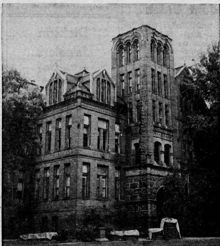
PIGEONS ARE HOMELESS with the removal of the administration building tower, which was done this summer as a safety precaution. Besides taking the tower off, various improvements are being made in the building as part of a campus-wide betterment program.
