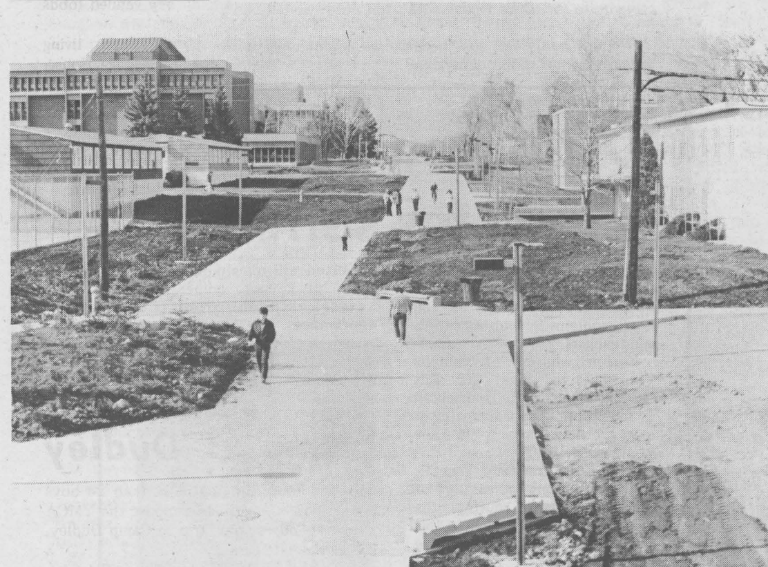
CAN YOU believe it? The above first picture was taken last fall in the midst of campus construction and lots of mud. The bottom picture was taken just recently, which shows
