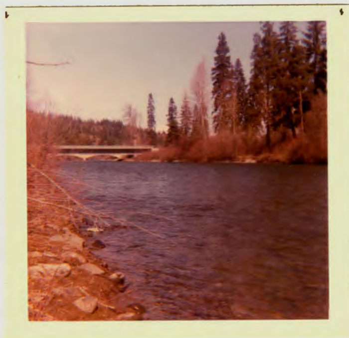
Fig. 6. Site IV, upstream view (March, 1971).
