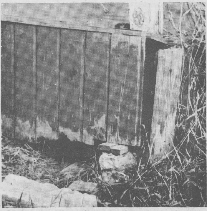
SHAKY FOUNDATION --One landlord has refused to fix this problem and student tenants have propped it up as best they could. At left an inoperative sewer system is uncovered. The one inch black pastic pipe in the foreground now runs directly from the house toilet on to an open field behind the house.
