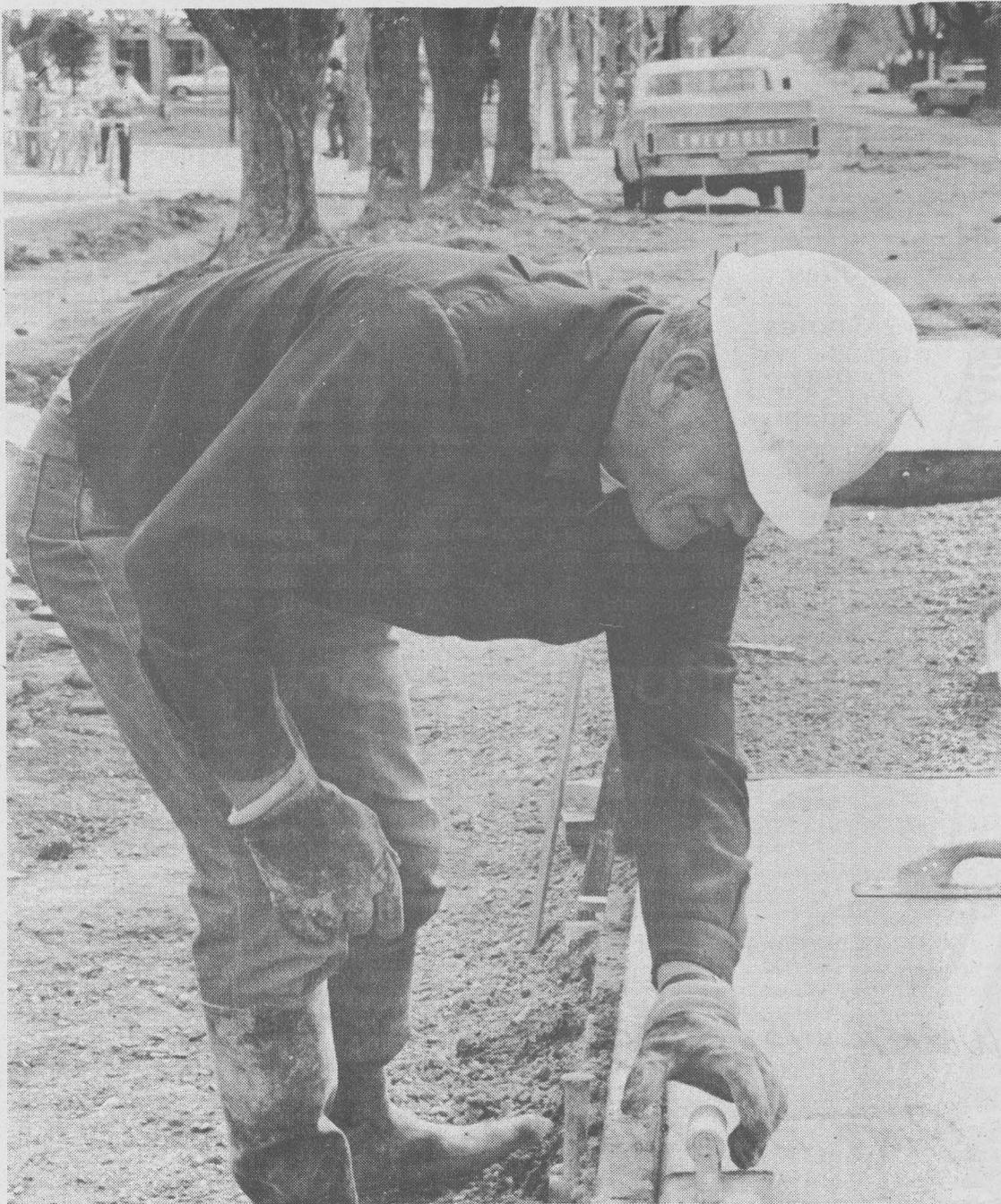
**REBUILDING THE MALL** has proven to be a slow, muddy, unsightly process. The South Campus Mall project is scheduled to be completed this biennium, and workmen are laying concrete now, as most underground work has been completed. Workman, Ken Sandifer, smooths the concrete walkway portion laid this week. [photo by Peter B. Mead]
