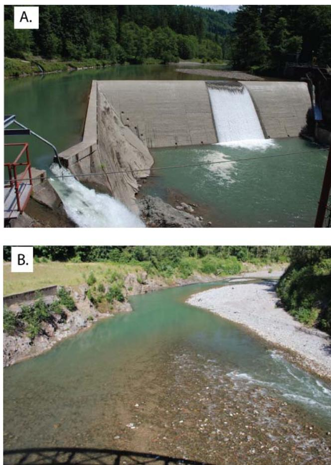
Figure 1: Images of Marmot Dam before and after removal. A: Former Marmot Dam, photo taken in 2007 (photo courtesy of Portland General Electric). B: Site of the former Marmot Dam site in the foreground, looking upstream toward the emptied reservoir in the background (photo taken by Carl Matzek)
