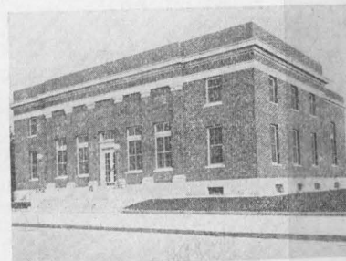
New $65,000 Federal Building.
