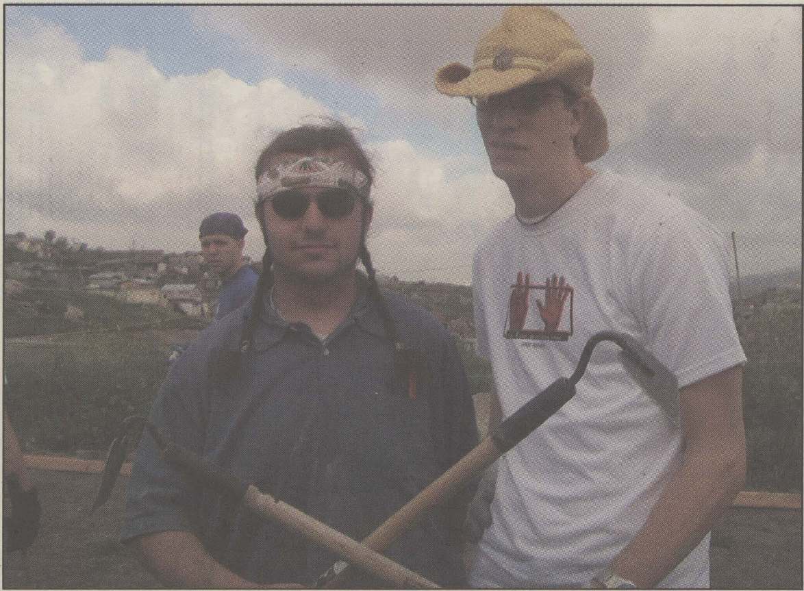
Aronica and Nathan Rains build a house in Mexico during Spring Break 2005.
